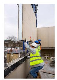
Small labour team required to construct 9 m long PSF wall
