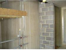
Blockwork and other finishes seamlessly integrate with PSF
