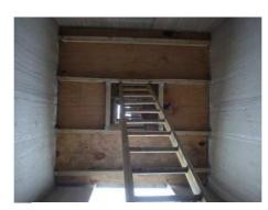
Safe internal access via hatches – removes need for scaffolding or external access tower in lift shafts
