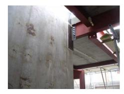
Steel frame can be directly attached to PSF walls
